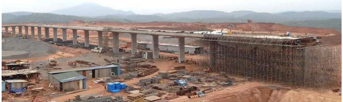
17 May, 2016 | Construction of Flyover
